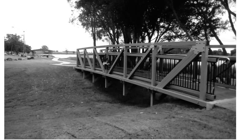
New Corcoran Park Bridge 10 Dorothy Cox
